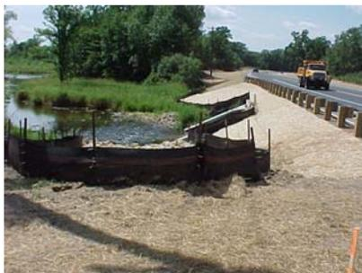
*Temporary cover and silt fence work together to prevent the discharge of sediment from this construction site.*
