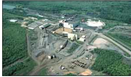
Stormwater retention ponds help this company manage runoff.
